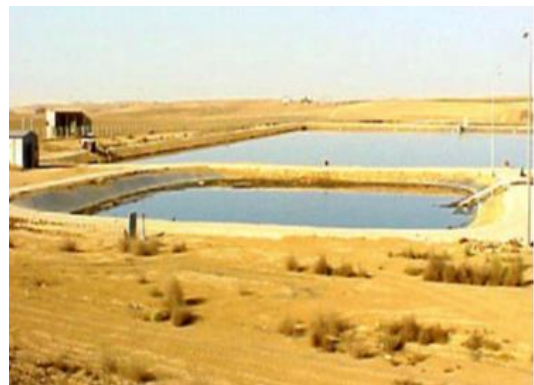
Fig.3 Anaerobic pond lined with a plastic membrane
